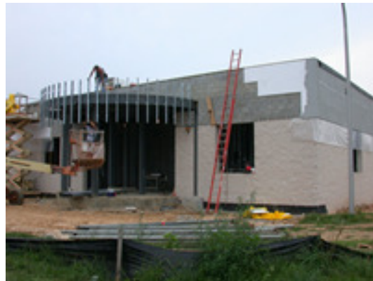
View of outside of facility during construction in 2003.
